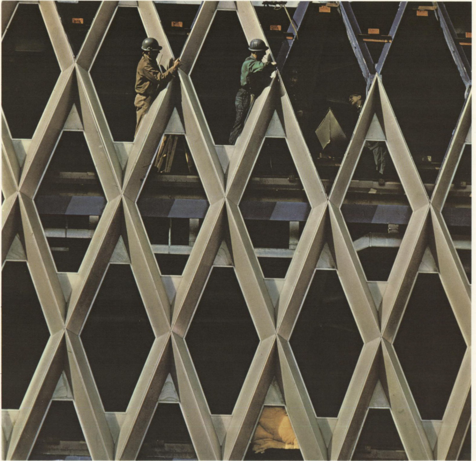
Construction workers installing the stainless steel exterior of a 13-story building that will house IBM's new branch office in Pittsburgh.
