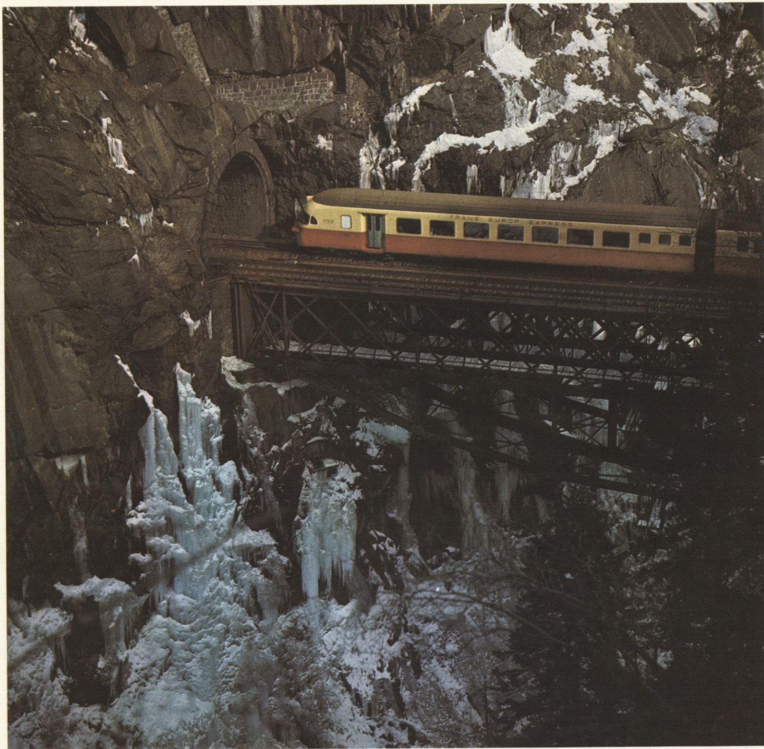
Swiss Federal Railways' express racing through the Alps. SFR uses IBM data processing systems to solve problems ranging from train scheduling to traffic forecasting.
